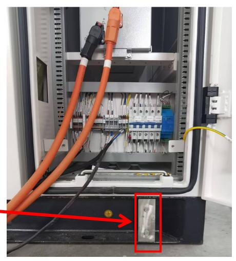
户外柜可用 2AWG 接地线(客户自供),M6\*16 接地螺钉,在每个柜体下方配备有接地孔,户外柜通过接地线接至现场接地系统。 Outdoor cabinets can be used with 2AWG grounding cable (supplied by the customer), M6\*16 grounding screws, and grounding holes are equipped under each cabinet, and the outdoor cabinets are connected to the on-site grounding system through the grounding cable.
