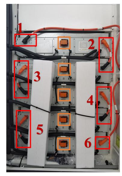
1、对应好正负极,由负至正依次连接,不可从正负两端开始最后连接中间,按图上 1、2、3、4、5、6 顺序连接。 Match the positive and negative terminals correctly. Connect in order from negative to positive. Do not start from both ends (positive and negative) and connect the middle last. Follow the connection sequence as shown in the diagram: 1, 2, 3, 4, 5, 6.
